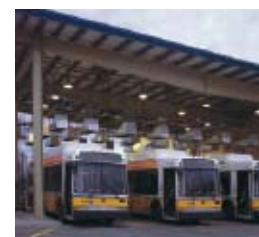
TRANSIT BUSES CLUSTER TO FUEL BY THE HUNDREDS OVER NIGHT, SUCH AS AT THIS CLEAN ENERGY STATION FOR THE MBTA SERVING GREATER BOSTON.
