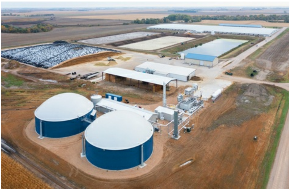
Clean Energy Renewable Natural Gas (RNG) Production Facility, Victory Farms Dairy, South Dakota. (Photo: Business Wire)
