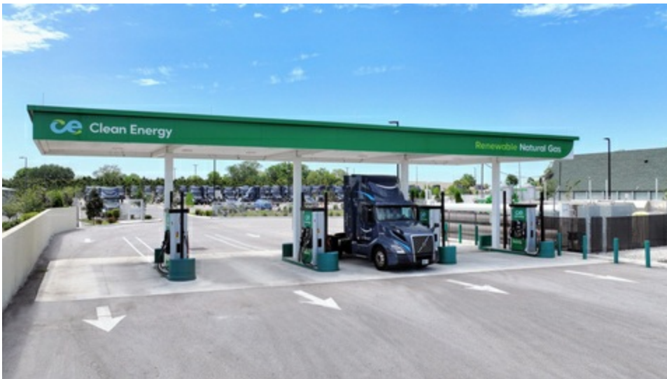
Clean Energy's new renewable natural gas (RNG) fueling station in Davenport, Florida. (Photo: Business Wire)
