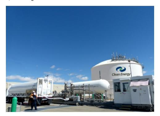
LNG loaded onto an ISO container at Clean Energy's liquefaction plant in Boron, Calif., for transport to Hawaii Gas in Honolulu, Hawaii. (Photo: Business Wire)
