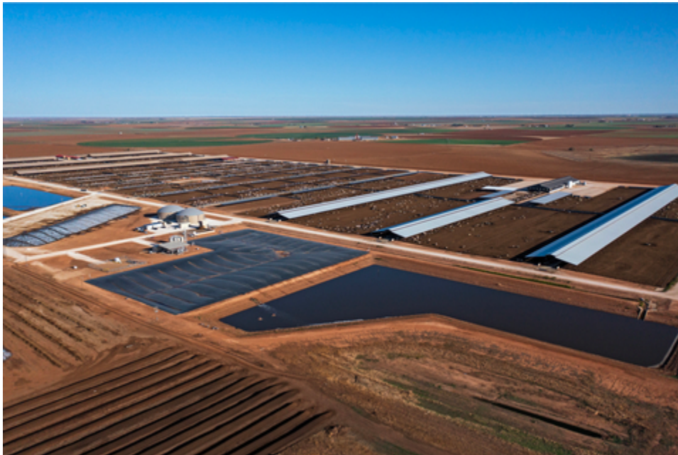
Del Rio Dairy (Photo: Business Wire)
