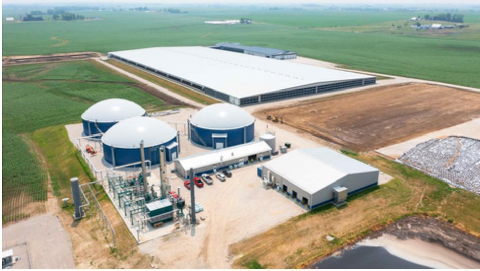
The three-digester facility located in State Center, Iowa, is now producing pipeline quality RNG and injecting it into the national grid. RNG is a sustainable fuel derived from organic waste that provides an immediate and significant carbon reduction in transportation.
