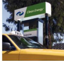
Small CNG fueling station
