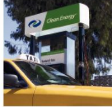
Small CNG fueling station
